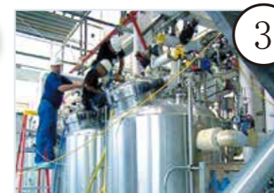
Process & Utility installations
