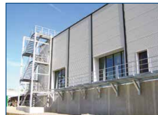
Vaccine filling plant, GlaxoSmithKline, Belgium
